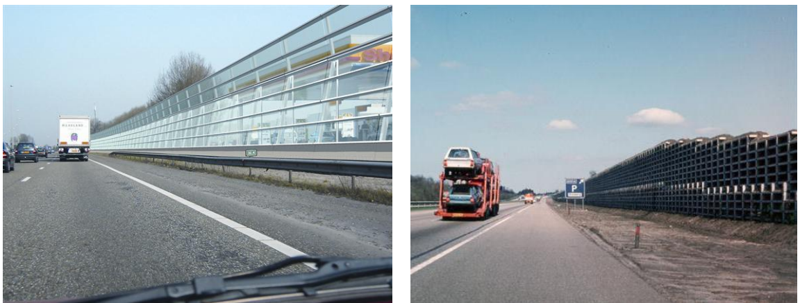
figure 27 Examples of noise barriers in the Netherlands (photos: beeldbank.rws.nl)
